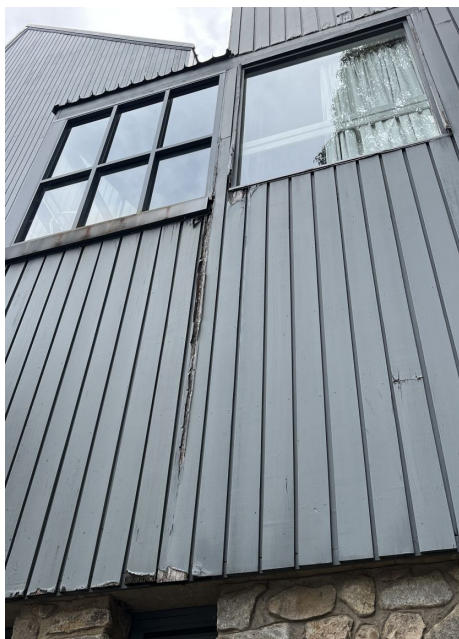
Figure 5 Windows on main entrance side of hotel, above carpark, note cladding deterioration particularly around window sill, and exposed bottom edge. Source: Kosciuszko Thredbo Pty Ltd, 22.02.22
