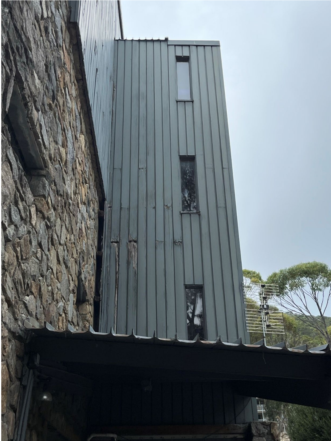
Deteriorated cladding above the maintenance workshop
